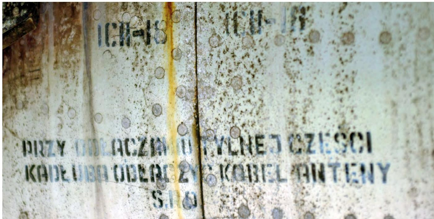
Stencilling on F1118 betrays its Polish origin; construction number 1C-1118 was visible at several places on the airframe. (23 August 2009, Marco Pennings)
